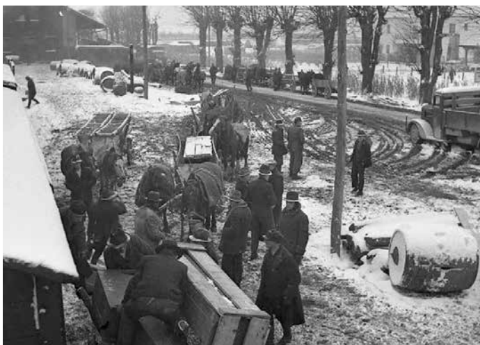
Cargo loading at the Gottschee train station
